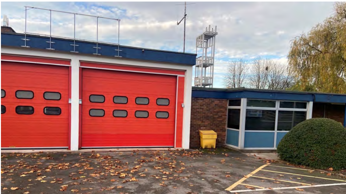
Knutsford Fire Station
